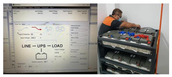
PS Systems are vital in our growing IT sector. They keep our servers and network infrastructure running 24/7 regardless of interruptions in power supply. As such, it is very important to be able to design and size a UPS system and also to verify its operation and capacity regularly.
